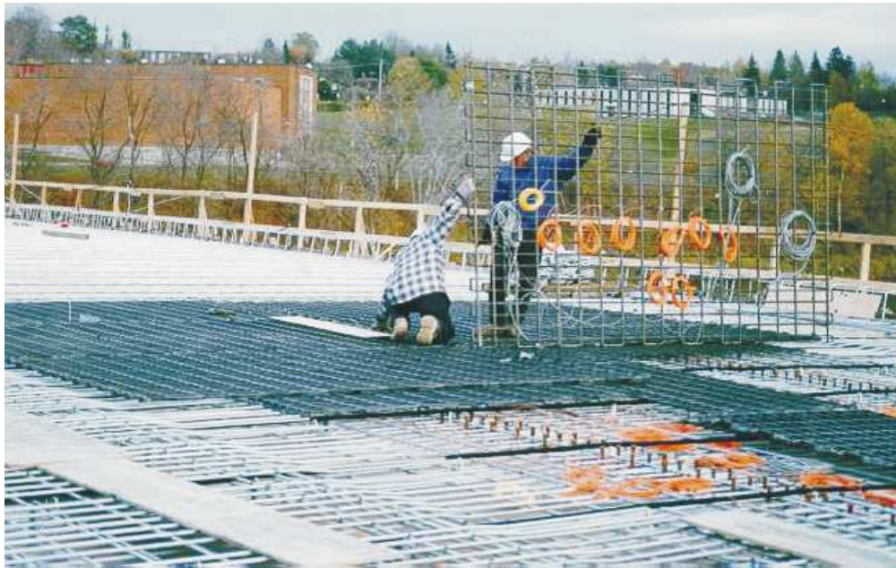
Fig. 10. Instrumented CFRP grid during the installation.
