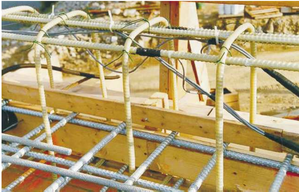
Fig. 8. GFRP reinforcement in the traffic barrier.
