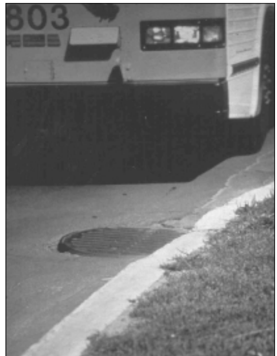
Figure 2. Vibrations are generated when a bus or truck strikes an irregularity in the road surface.
