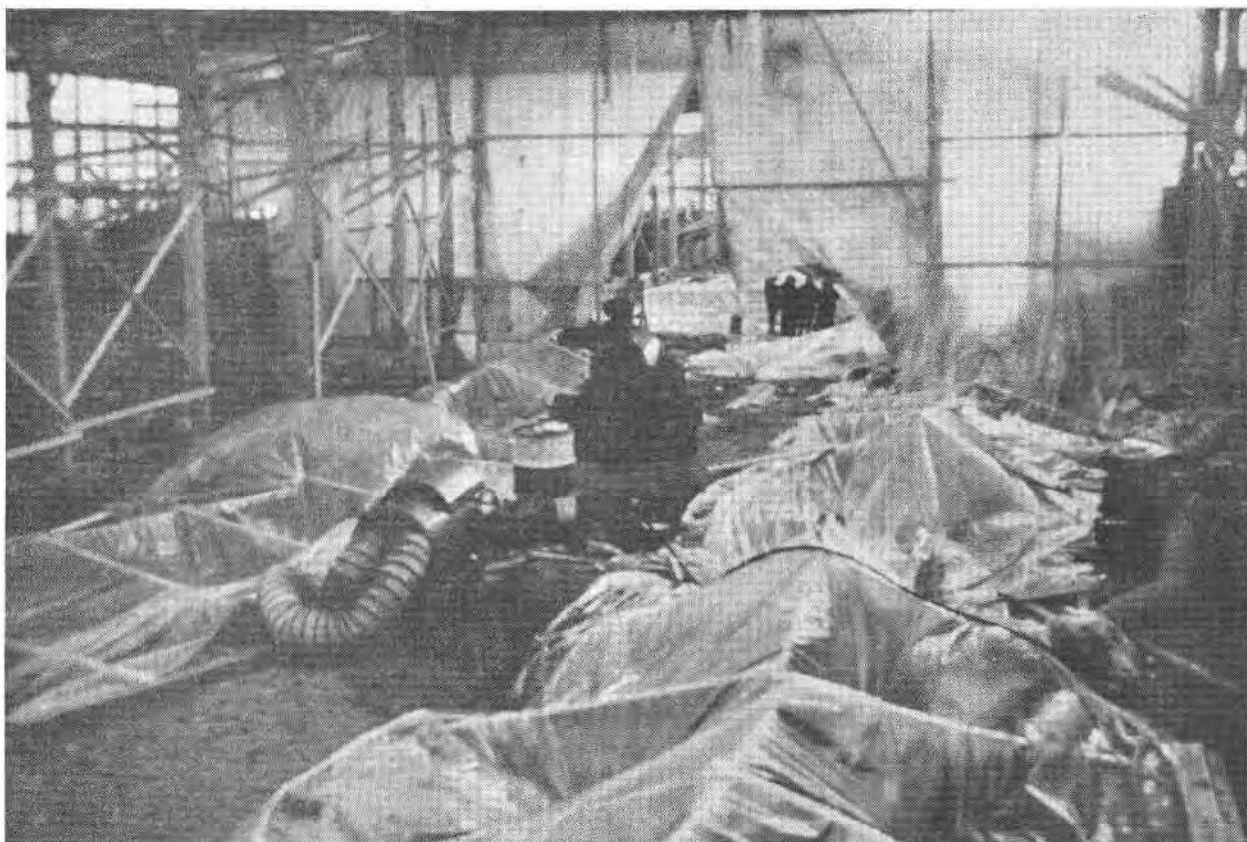
FIG. 5 Temporary enclosure, Fermont project (courtesy Pentagon Construction (1969) Co. Ltd.)
