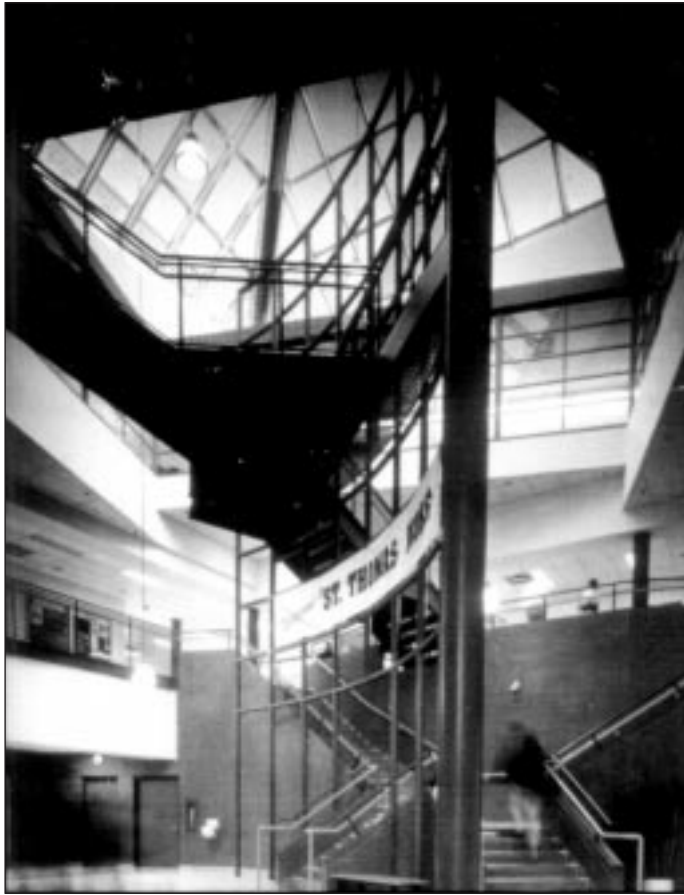
Figure 3. A recently built school in Hamilton, Ontario in which HSS columns filled with bar-reinforced concrete were used
