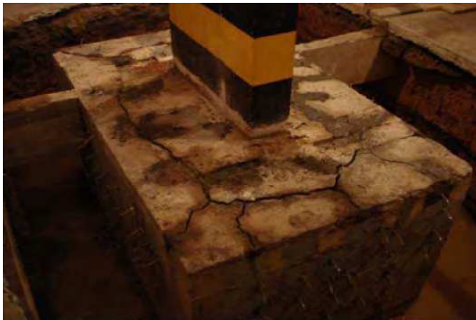
Figure 1. Building foundation with AAR-induced cracks under repair by epoxy injection (Andrade 2006).
