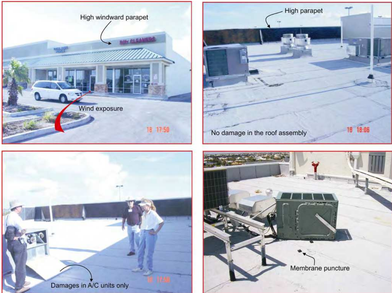
Figure 8: Survived roof assembly due to high Parapet and damages caused by the rooftop equipments.
