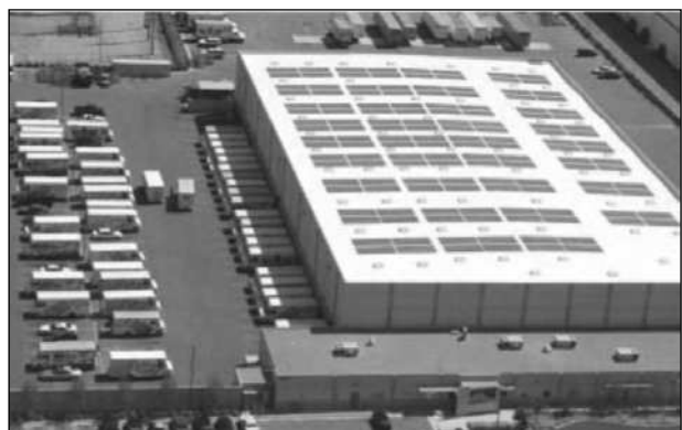
Figure 6. Integrated solar electric roofing system (flexible photovoltaic modules laminated on thermoplastic membrane) on Frito-Lay Distribution Facility, Los Angeles, California (Photo courtesy of Sarnafil Inc.)
