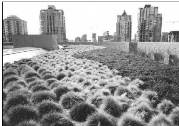
Figure 2. An intensive garden roof system (350-mm growing medium planted with ornamental grasses) on the Vancouver Public Library in Vancouver
