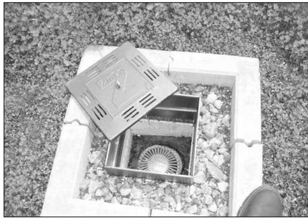
Figure 4. Roof drains on garden roof systems should be easily accessible and regularly inspected to ensure proper drainage. (Photo courtesy of Hydro-Tech Membrane Corp.)
