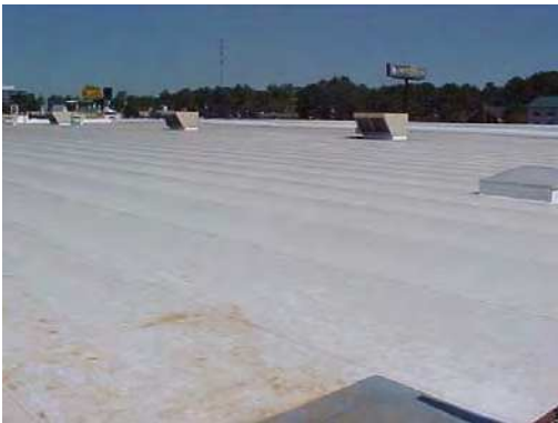
Figure 3. Billowing of a mechanically attached roofing system
