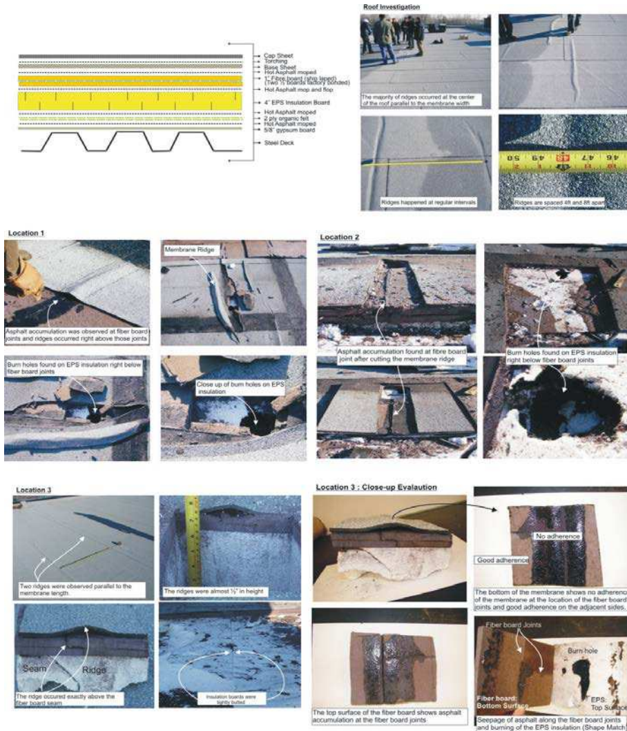
FIGURE 2: INVESTIGATION OF SCHOOL ROOF IN MONTREAL: CASE STUDY 1
