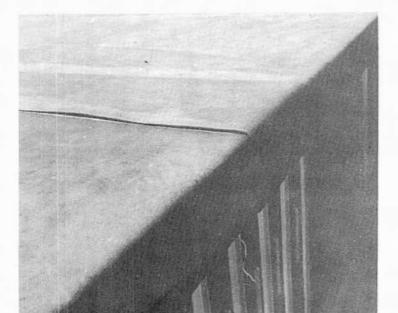
ROOF NO. 3 - 5 years exposure: colour change, chalking and adhesive failure.
