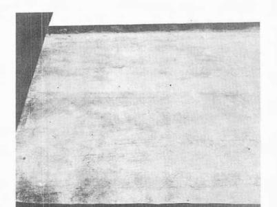
ROOF NO. 9 - 5 years exposure: membrane cracked, severe surface erosion, and heavy dirt retention.
