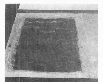
ROOF NO. 6 - 5 years exposure: heavy dirt deposition and surface erosion.
