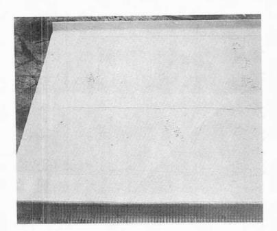
ROOF NO. 1 - 5 years exposure: severe hairline cracking.
