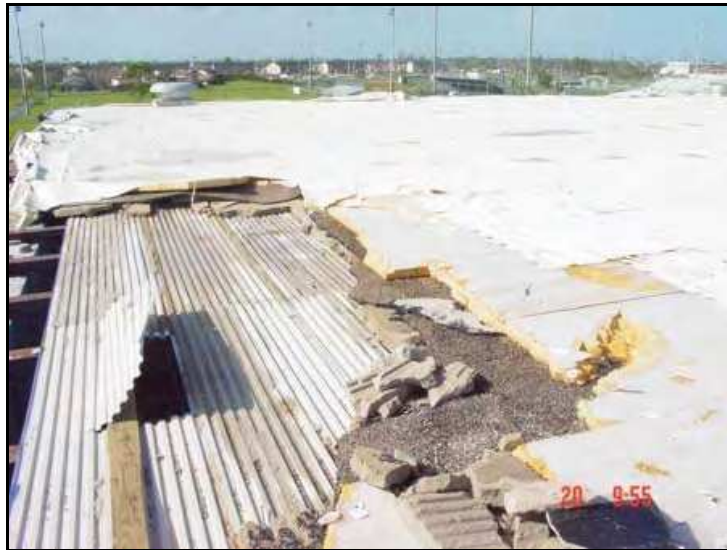
Figure 1: Roof damage during a high wind event
