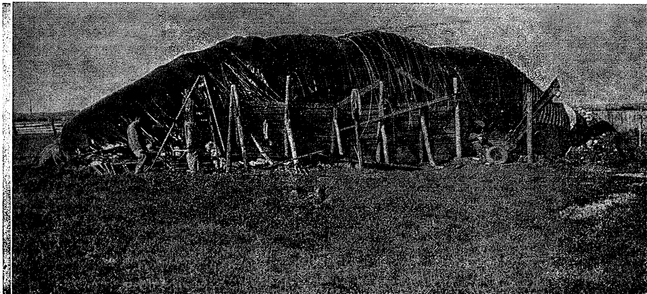
Fig. 1 (a) General view of collapsed silo.
