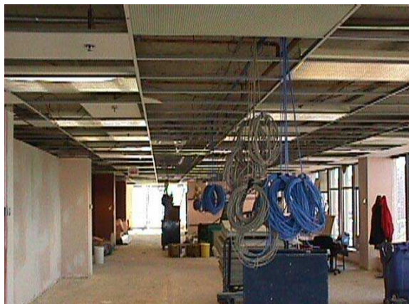
Figure 7. Cable installation in plenum space.
