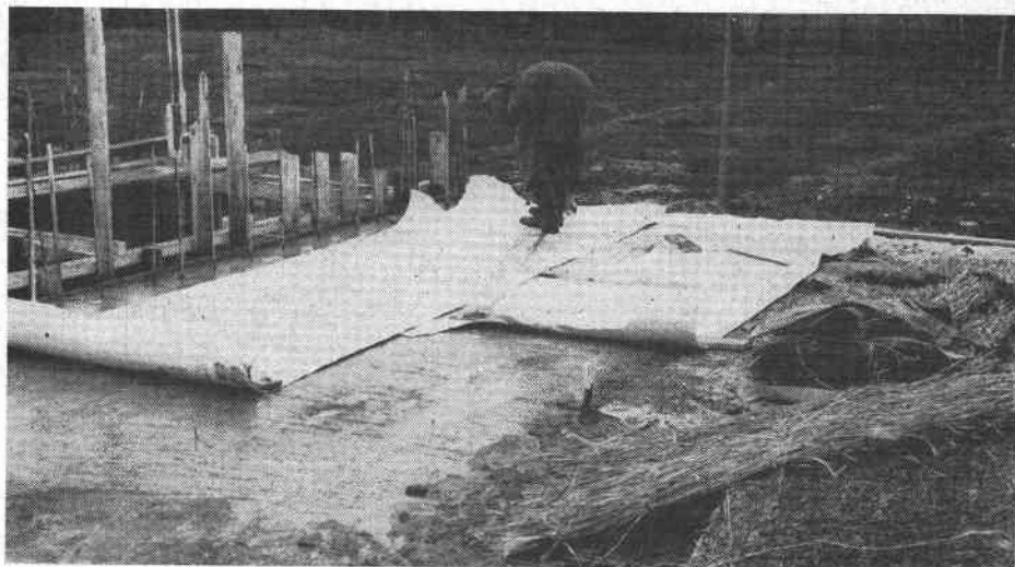
Fig. 2—Covering green concrete with knot pulp board and straw mats
