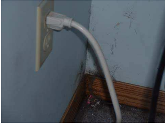
Mould on walls, at corners of floor and ceilings
