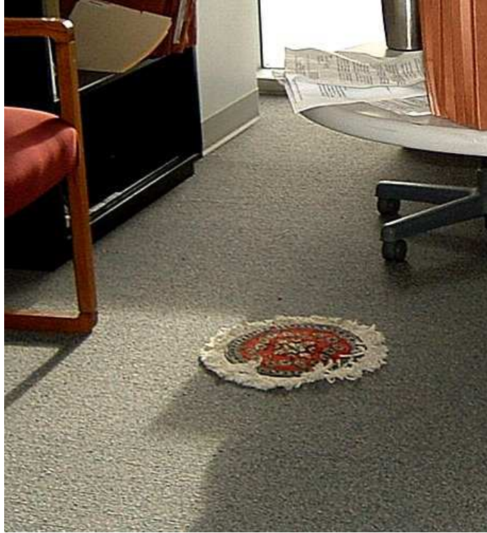
Figure 1. The underfloor air distributions system in this building created unpleasant cold draughts. The occupants reacted by covering the vent with this attractive carpet!
